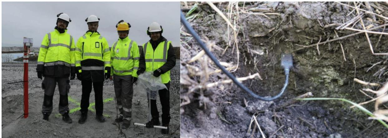
**Figure 2.** IoT soil moisture sensor installation. In the left image, the soil moisture sensor is attached to the wooden pole, and in the right image, the probe is situated 5 cm below the surface of the ground.
